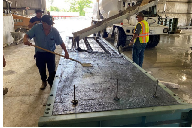
f) Casting of UHPC materials in form
