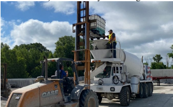
c) Loading of water and water reducer
