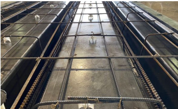
a) Forms ready for casting
