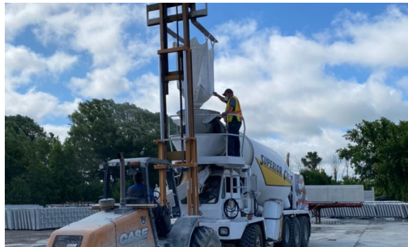
b) Loading of sand into ready-mix truck
