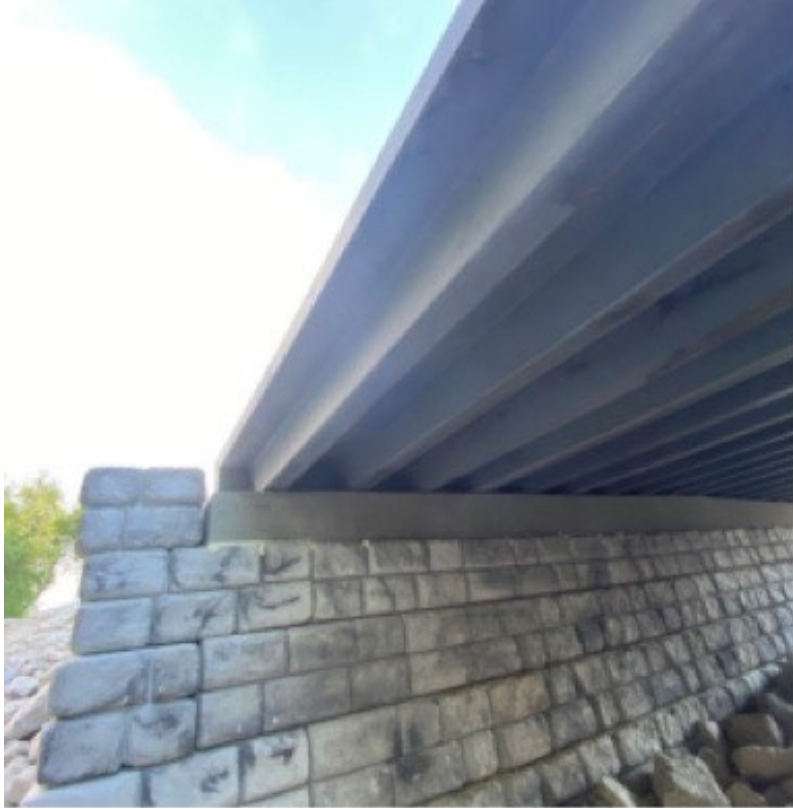
FIGURE 24: Close up of bridge superstructure (picture courtesy of William Hazelton)
