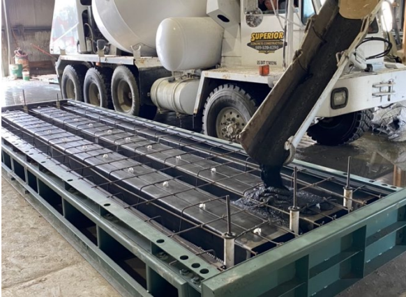
e) Casting of UHPC materials in form
