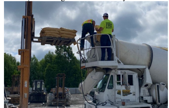
d) Loading steel fibers
