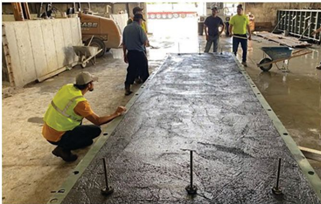
Figure 3. Fabrication of ultra-high-performance concrete (UHPC) ribbed panels.
