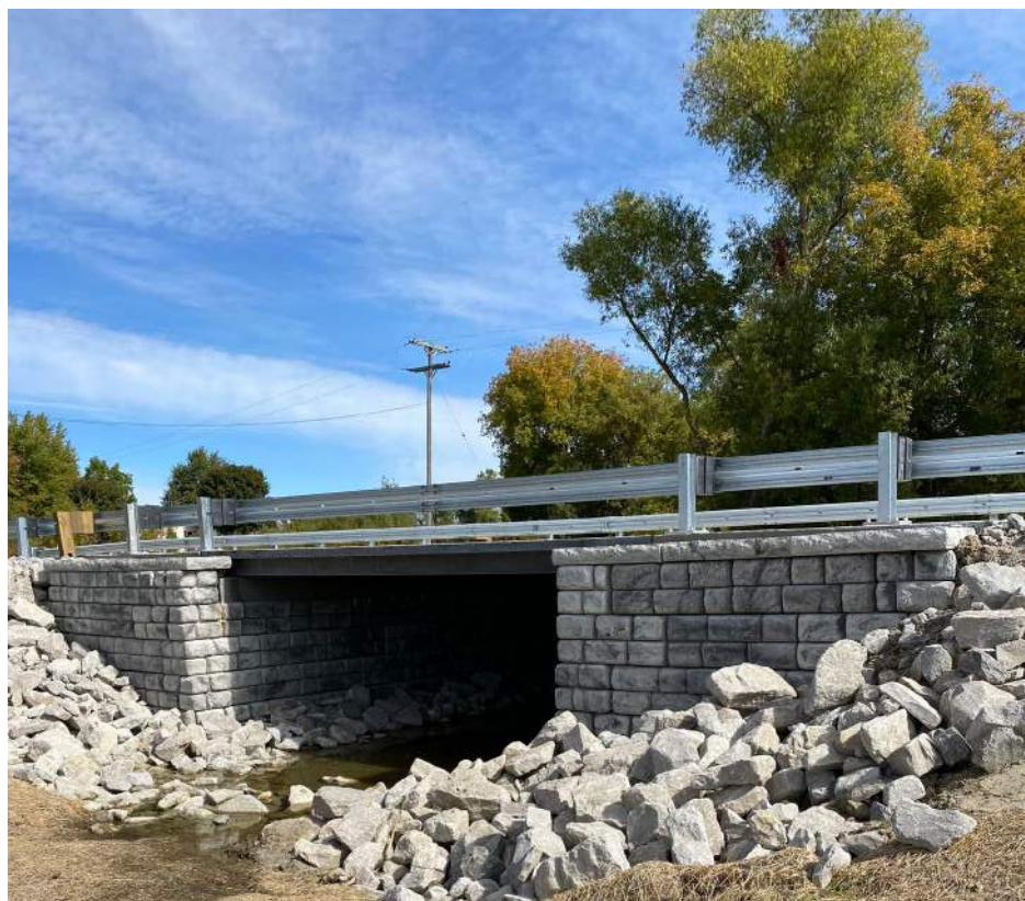
Figure 6: Finished Bricker Road Bridge over the Quackenbush Drain
