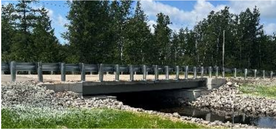
Figure 3: Finished UHPC/PBTG bridge system: Mostetler Road over Mostetler Creek Bridge
