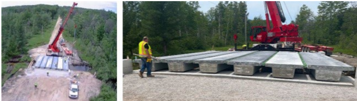
Figure 2: Construction process of the UHPC/PBTG bridge system
