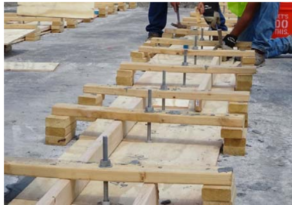
(b) Top forms after placement
