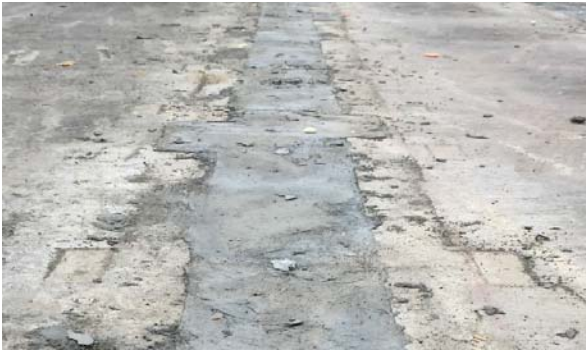
(a) Poured UHPC connection
