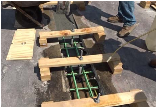
(a) Pre-wetting and placement
